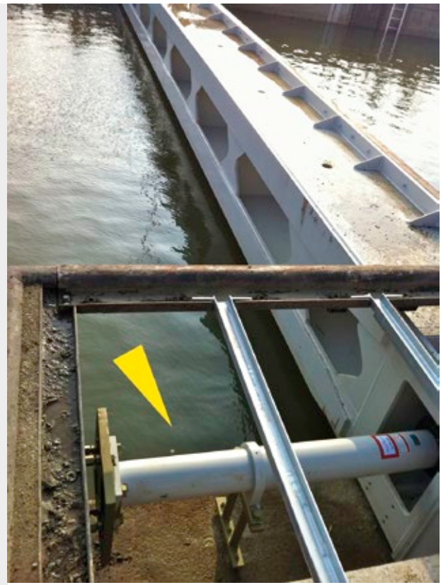
Heavy safety shock absorbers, which are specially designed for this application, are able to brake in lock masses of up to four million kg Mourik Limburg BV, 6101 AJ Echt, Netherlands
